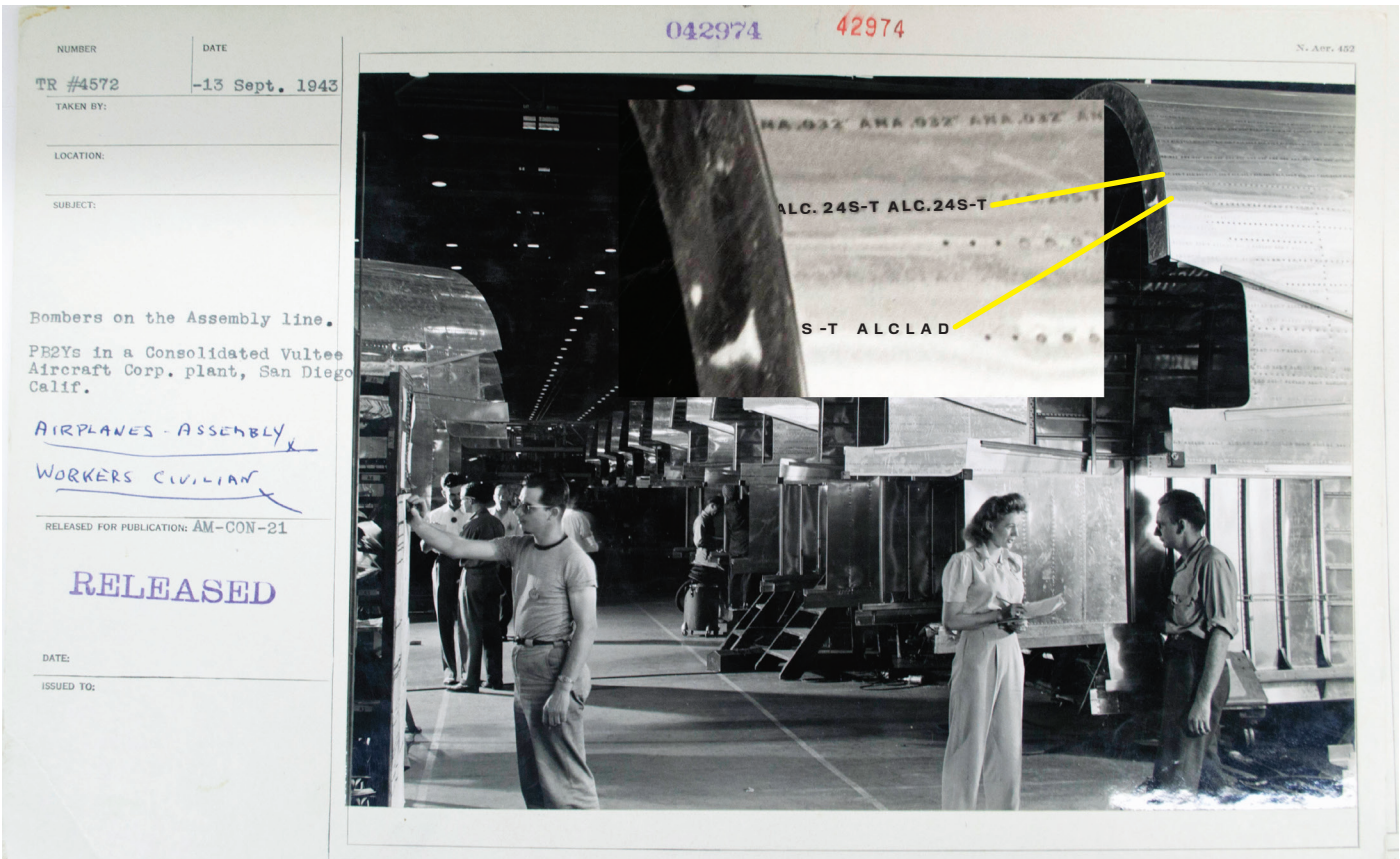
PB2Ys under construction, with inset detail.
