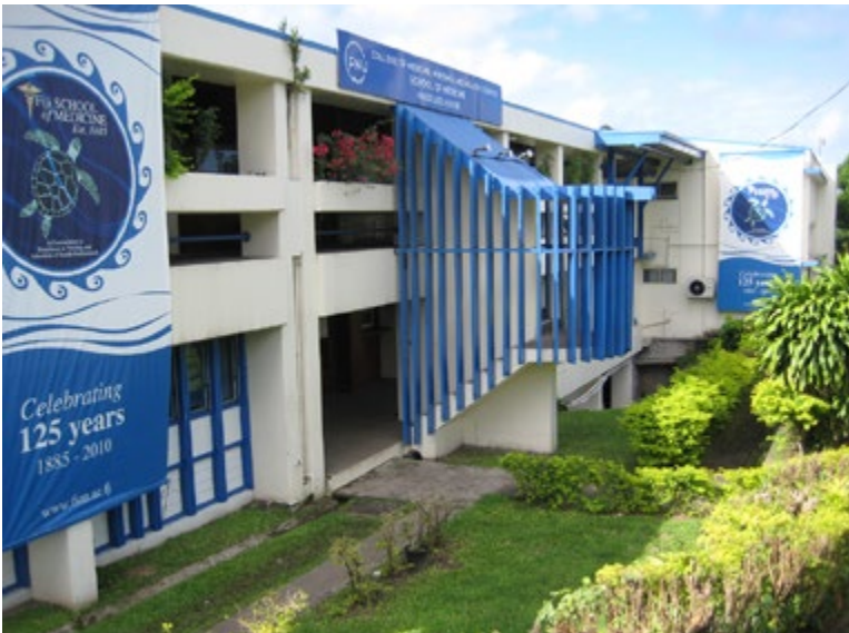
Hoodless House Office/Classroom Building. Photograph by Gary F. Quigg.
